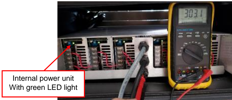
Figure 9: Back side of ROV Power Supply
